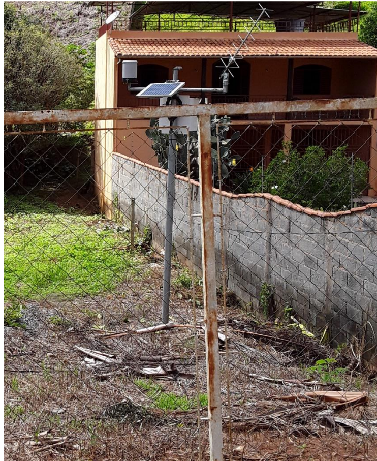
Figura 80 – Painel de controle – Rua Nova 2
